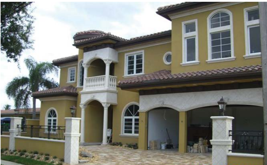
Photo courtesy Safe Harbor Design/Build
